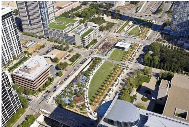
Figure 9: Klyde Warren Park, Dallas TX, is a cap park over the recessed highway
