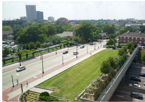
Figure 10: Fifth Street bridge, Atlanta GA, has large landscape edges that create a noise and visual buffer the interstate below, and integrate bike and bus lanes
