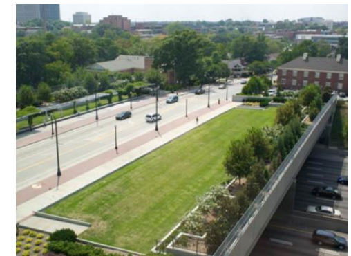
Fifth Street bridge, Atlanta GA, has large landscape edges that create a noise and visual buffer the interstate below, and integrate bike and bus lanes
