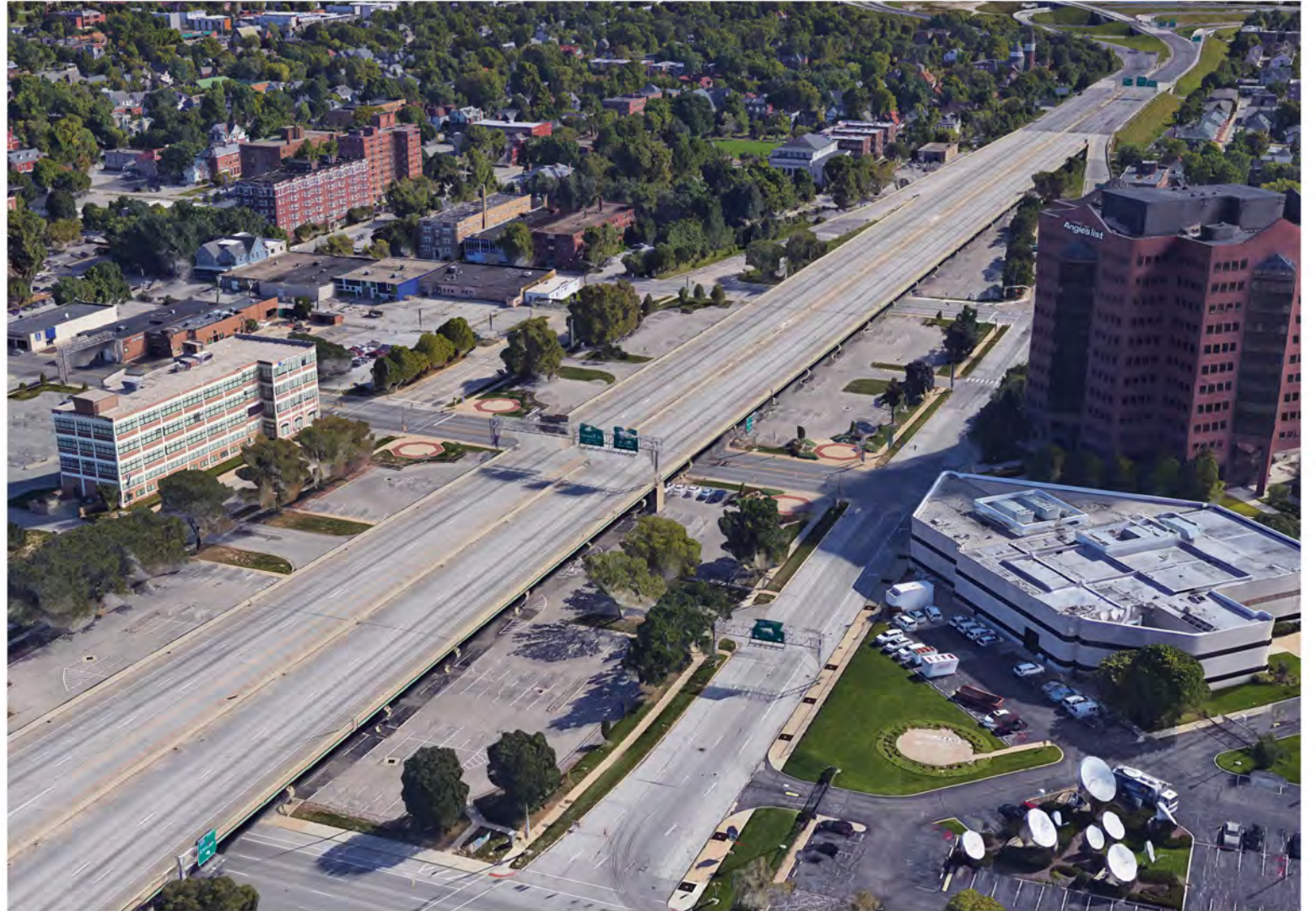
REBUILD AS-IS OPTION (above) Image location - Inner Loop, North Leg (I-65) Source: Google Earth
