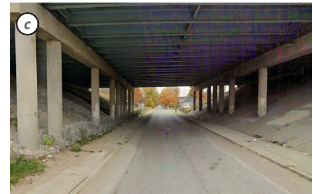
Naomi underpass [View east]
