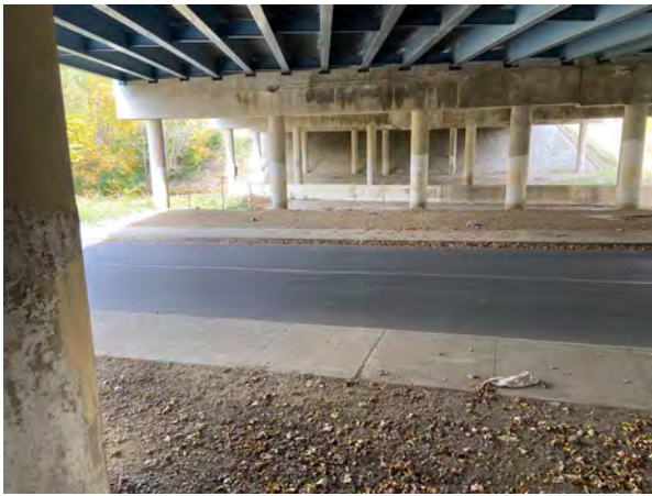
Nelson Avenue and Bean Creek Underpass
