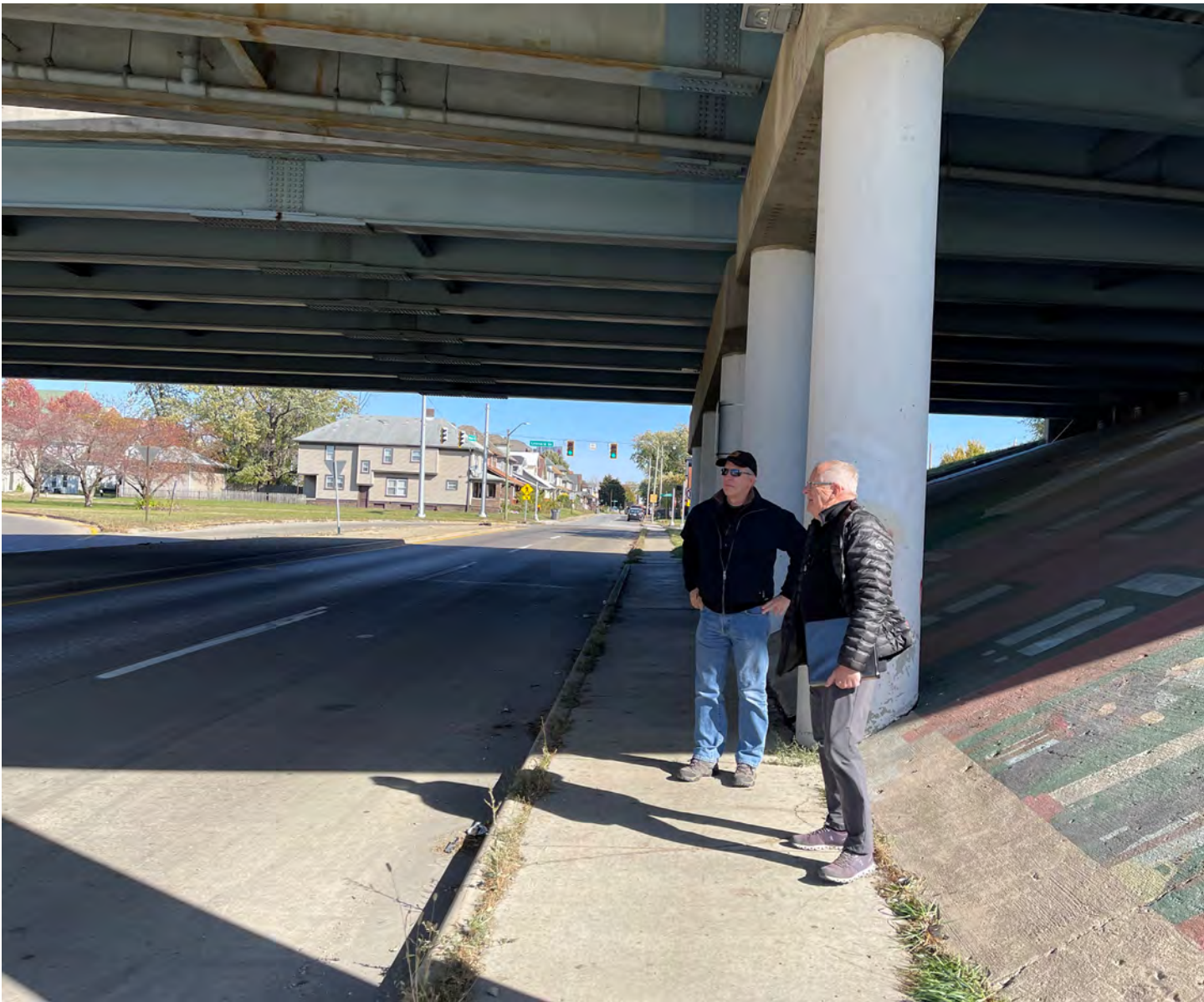
Rethink advisors reviewing connectivity constraints at Morris Street on October 19, 2022. Site reconnaissance informed the recommendations included in this report.
