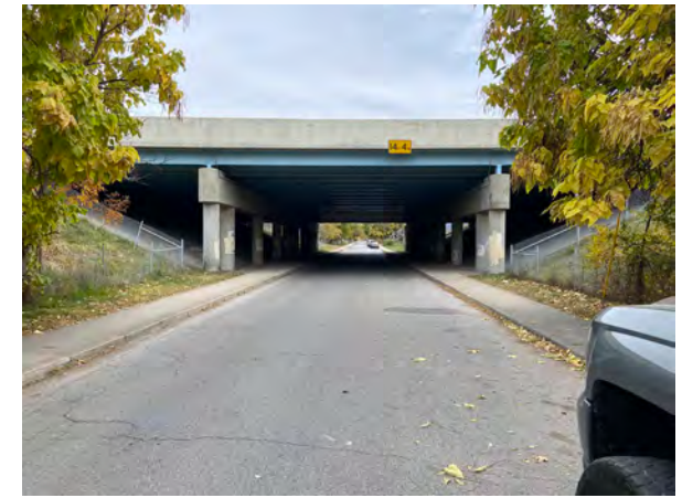
Bradbury Avenue Underpass
