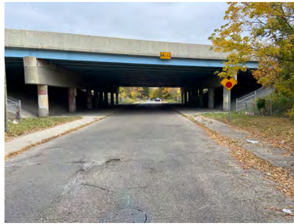
Southern Avenue Underpass
