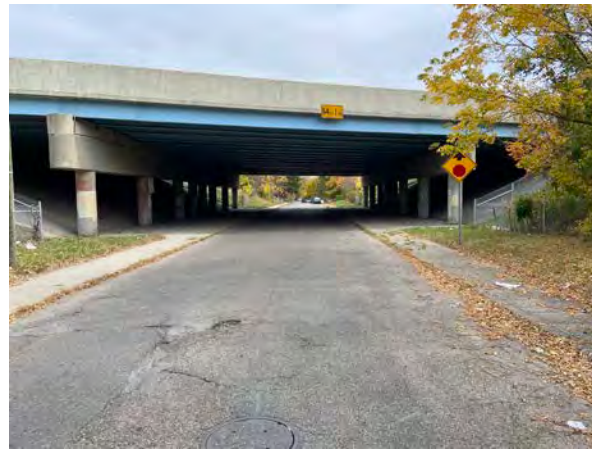
Southern Avenue Underpass
