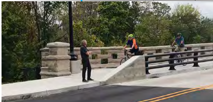
Central Bridge barrier rail along curb line showing end treatment. End treatment same at both ends and symmetrical both sides. If sufficient space is available the end treatment could also flare away from the roadway as shown in the diagram above. Speed limit on Central Avenue is 35 mph, same as Hanna Avenue.
