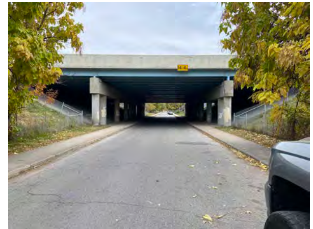
Bradbury Avenue Underpass
