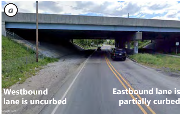
The SAFE project should address deficient underpass conditions such as this uncurbed narrow path to a school
