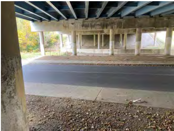
Nelson Avenue and Bean Creek Underpass
